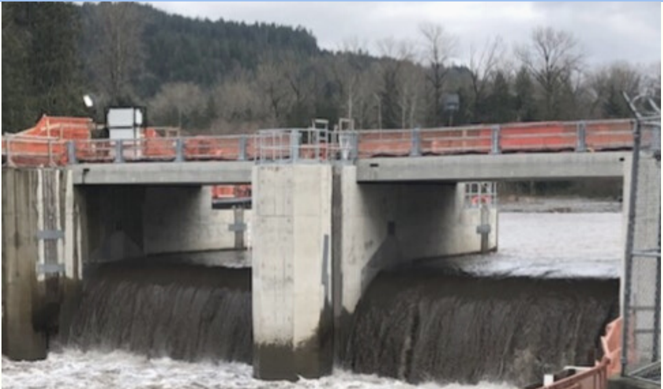
Obermeyer Gates at USACE Mud Mountain Dam Fish Diversion Used in Conjunction with Trap and Truck Operation
